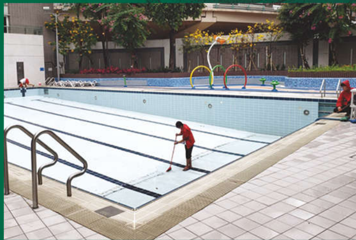
Annual Repair Work for the Swimming Pool 游泳池年度維修工作
